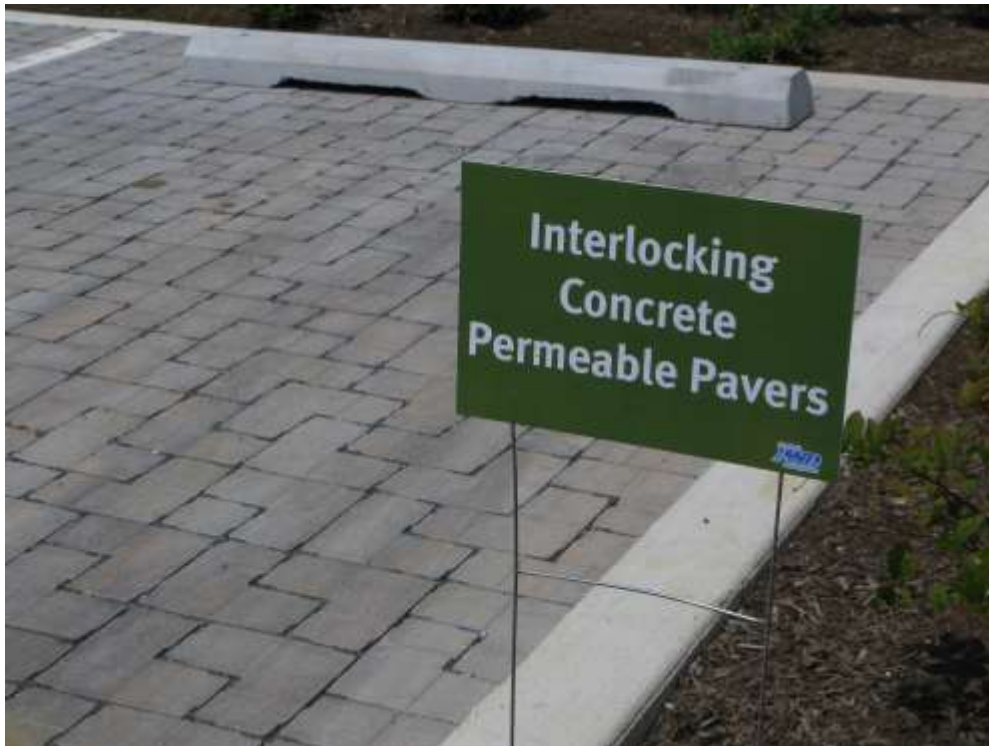
Figure 4-7 – Permeable Interlocking Concrete Pavers (source: EPA)
