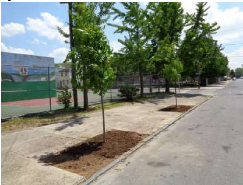
Figure 4-3 - Photo of Enhanced Tree Pits
