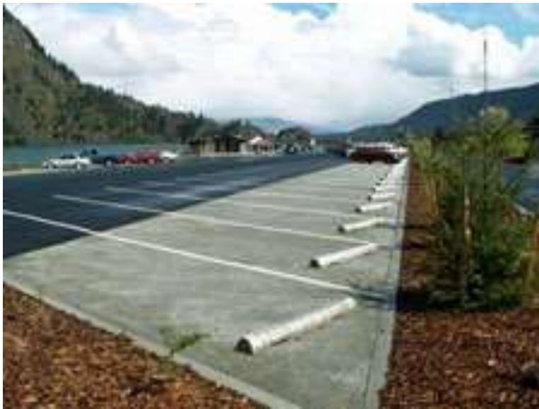
Figure 4-6 – Pervious Concrete Panels
