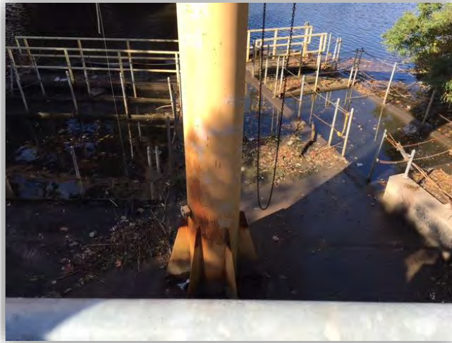
Photo No. 21 – Johnston Avenue Outfall During a Hide-Tide Period
