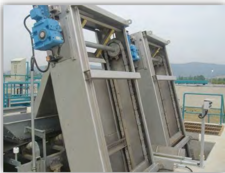
Photo No. 10 – Multiple Climber Screen Installation
