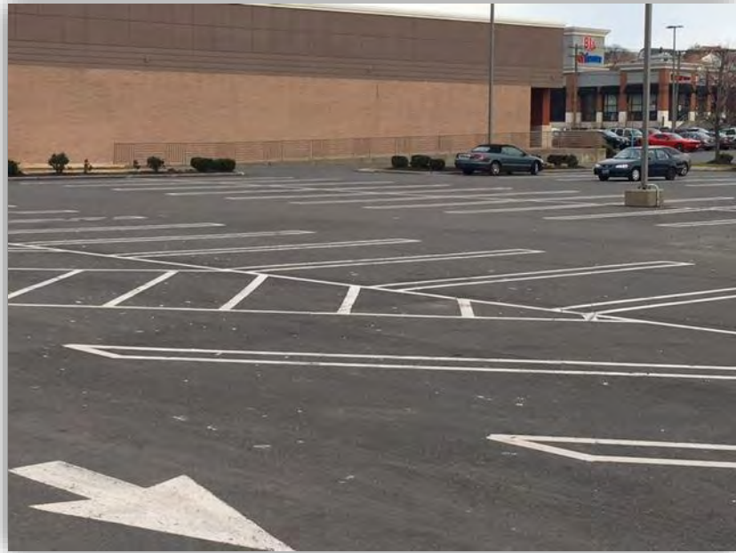
Photo No. 19 – Commercial Development in the Vicinity if the Nairn Avenue Outfall
