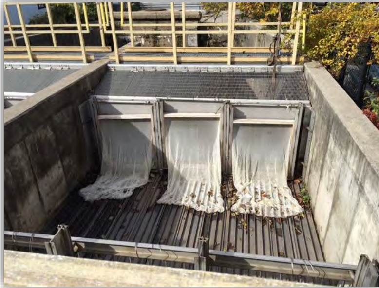
Photo No. 13 – Netting Chamber at Ivy Street Outfall
