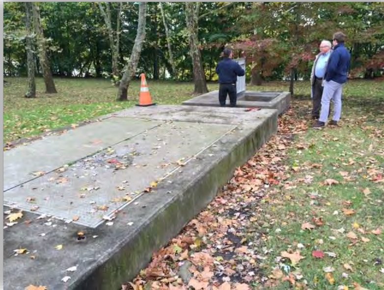
Photo No. 18 – Outfall Site KE 001 – Stewart Avenue
