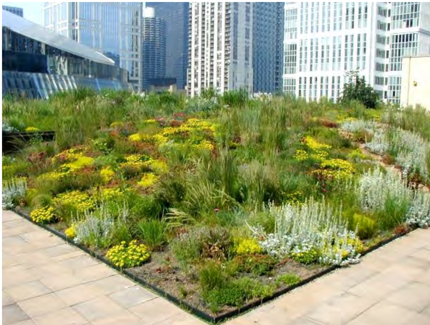
Figure 4-4 - Photo of Green Roof on Chicago City Hall
