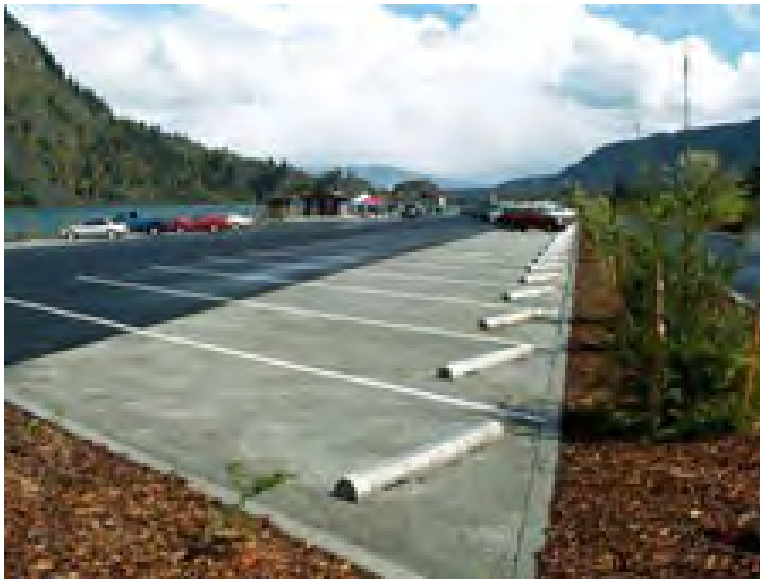
Figure 4-6 – Pervious Concrete Panels
