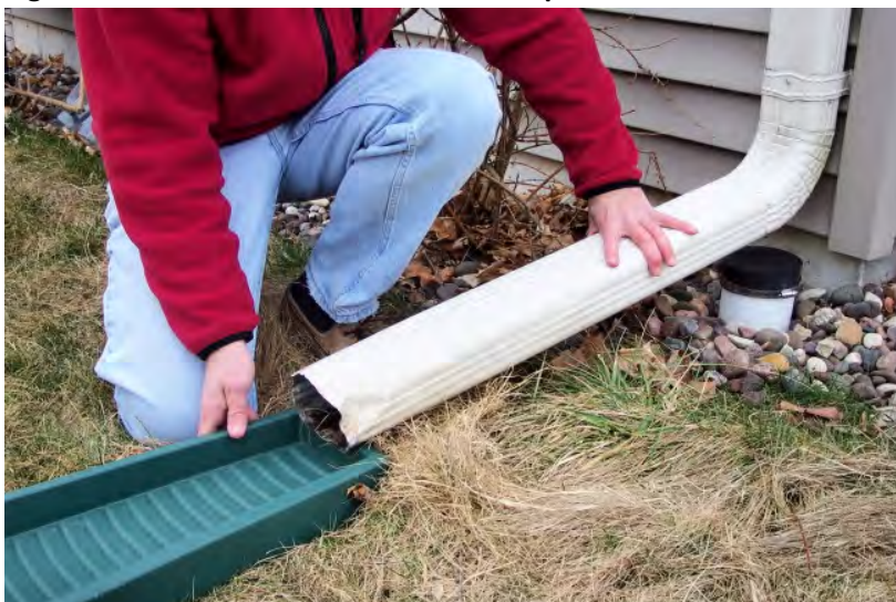
Figure 4-5 - Photo of Disconnected Downspout
