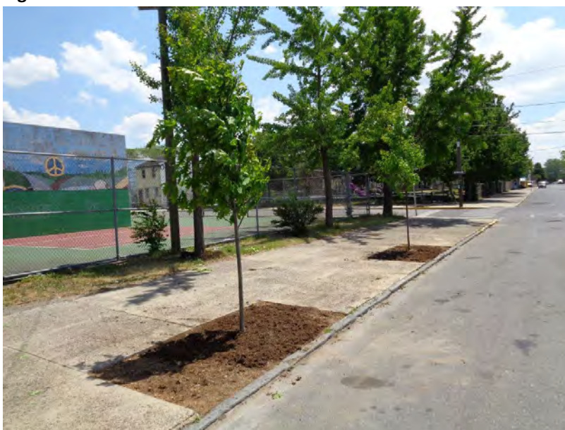
Figure 4-3 - Photo of Enhanced Tree Pits
