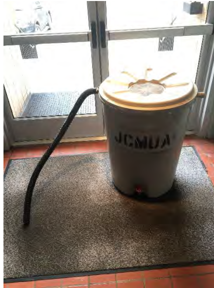
Figure 2-5: Typical JCMUA Rain Barrel
