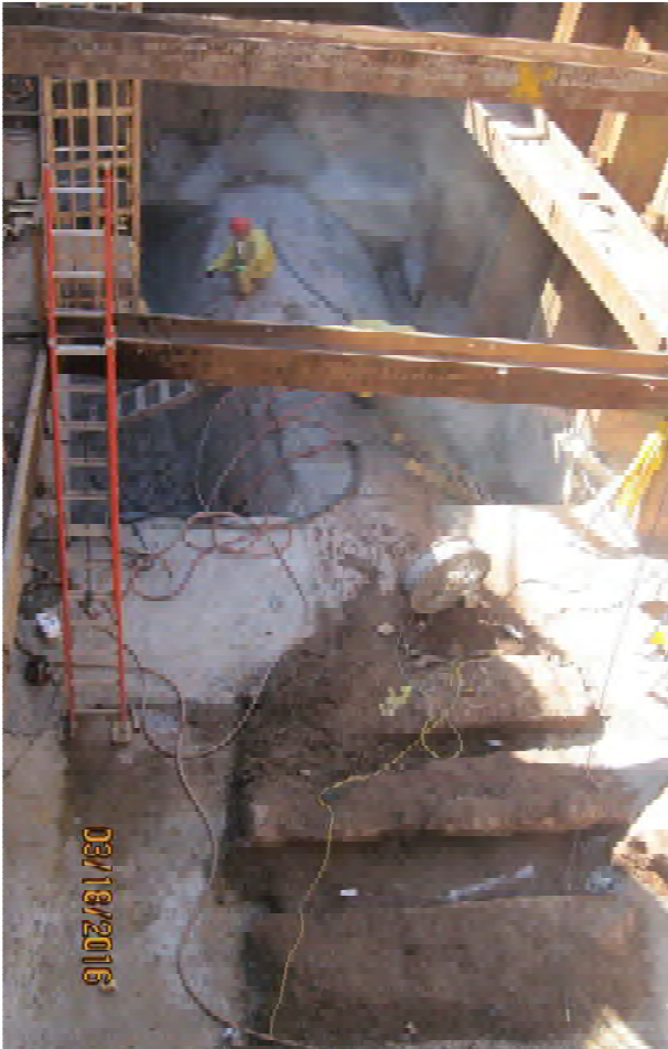
90" Diameter Main Interceptor State Street, Passaic
