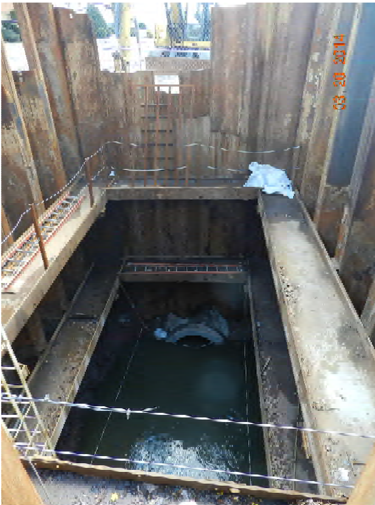
72" Main Interceptor Within Route 20, Paterson
