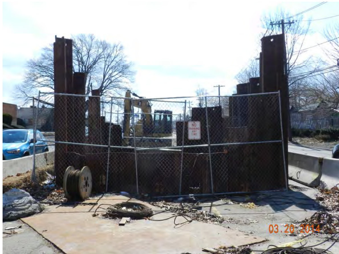
72" Main Interceptor - Within Route 20, Paterson
