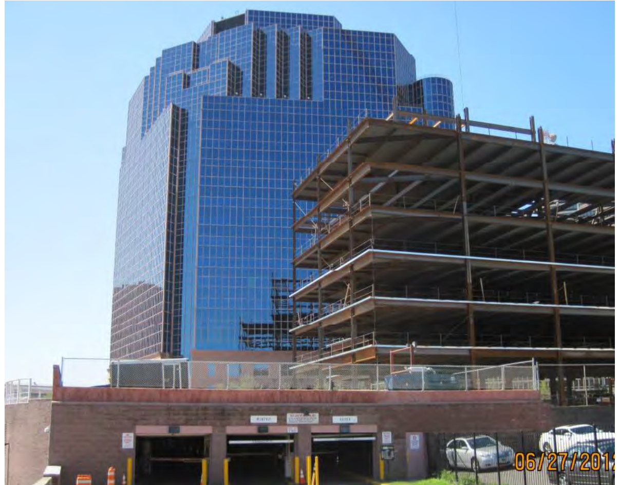
141" Main Interceptor - Beneath Panasonic Building, Newark
