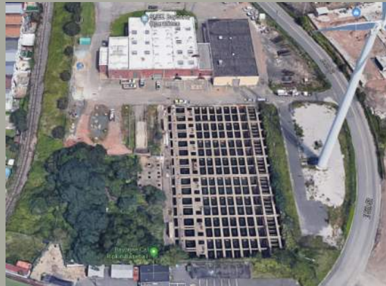
Existing storage tanks at Bayonne's E 5 th St Facility
