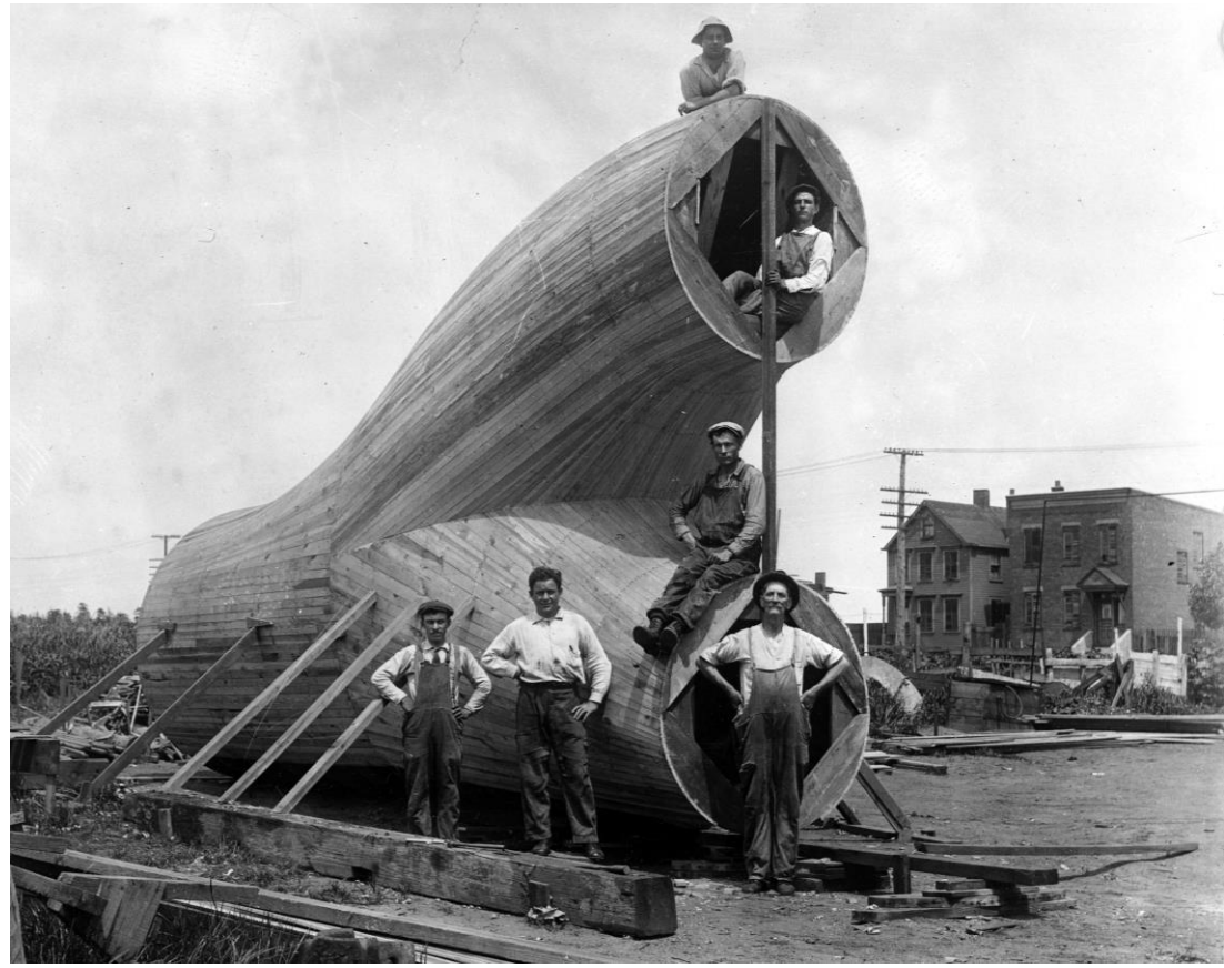
PVSC Interceptor Construction, 1920s
