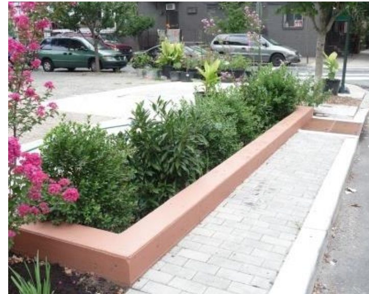
Stormwater Planter at Columbus Square
