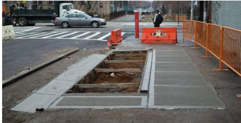
Engineer Soil Added
