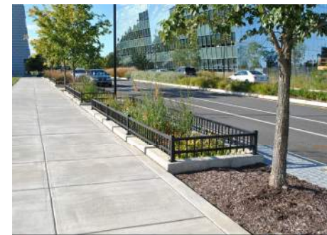
What is a "Greened Acre"? A Greened Acre manages at least the first inch of rainfall over an acre of hard surfaces. PHILADELPHIA WATER In other words, a single rain garden that can absorb an inch of rain from a one-acre parking lot would equal one (1) GA; a rain garden that can absorb one inch of rain from a three-acre parking lot equals three (3) GA.
