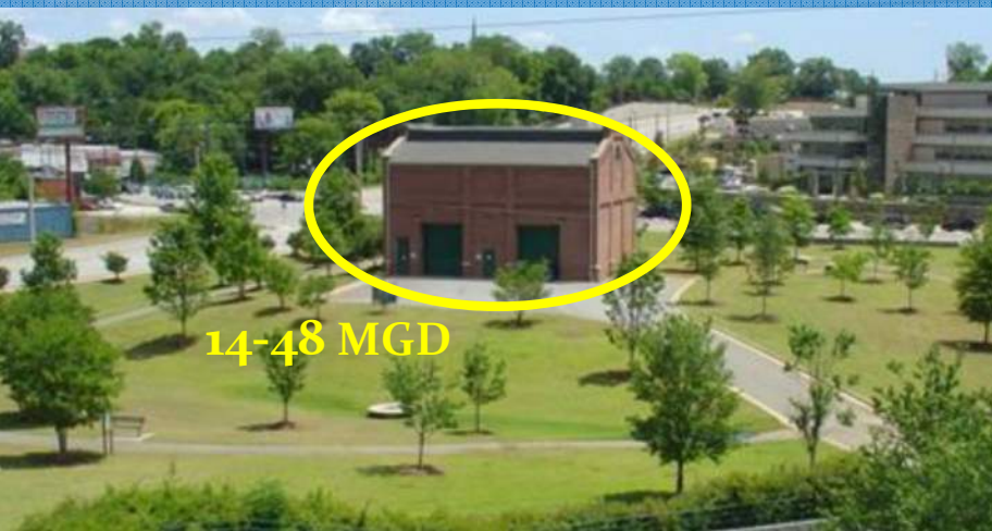
Uptown Park CSO Facility Columbus, GA
