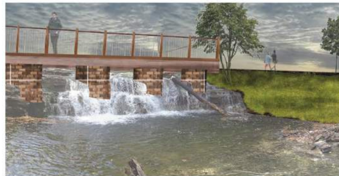
2. The pedestrian bridge over the canal showcases the weir that controls the flow of water from the Passaic River into the canal.
