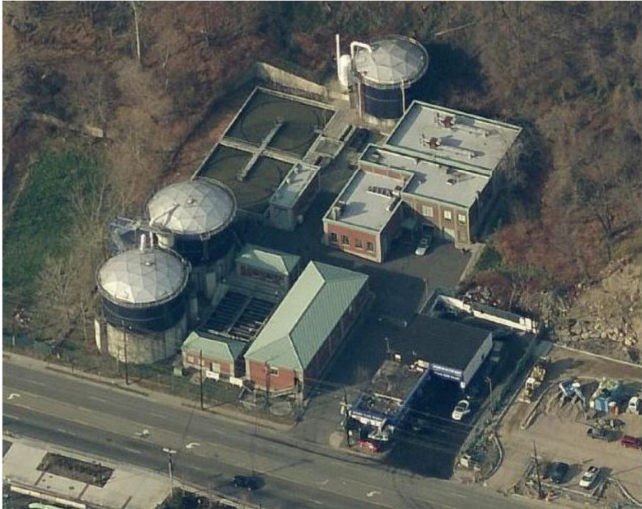
Figure C-1: The Woodcliff Sewage Treatment Plant
